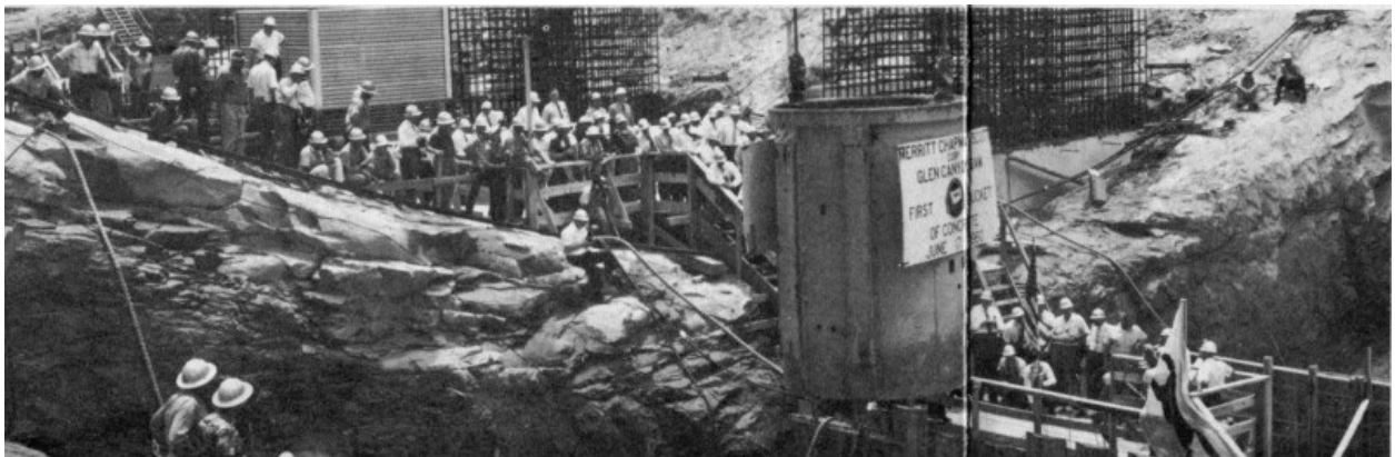
The first placement of concrete—June 17, 1960.
