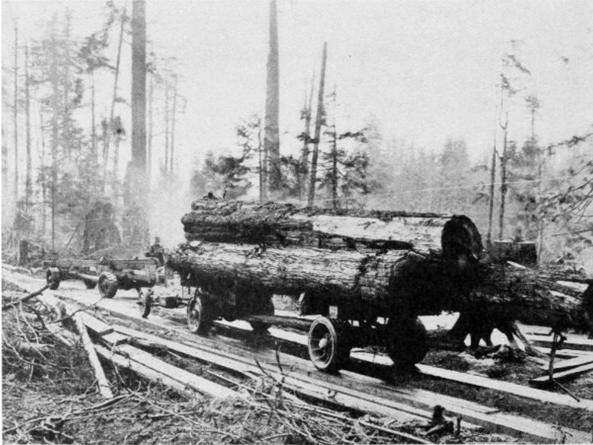
Turn out on fore-and-aft plank road.
