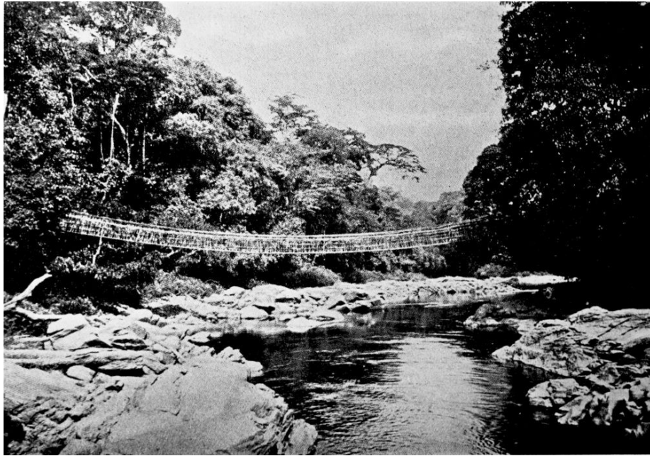
SUSPENSION BRIDGE OVER THE FI, NEAR TINTO.
