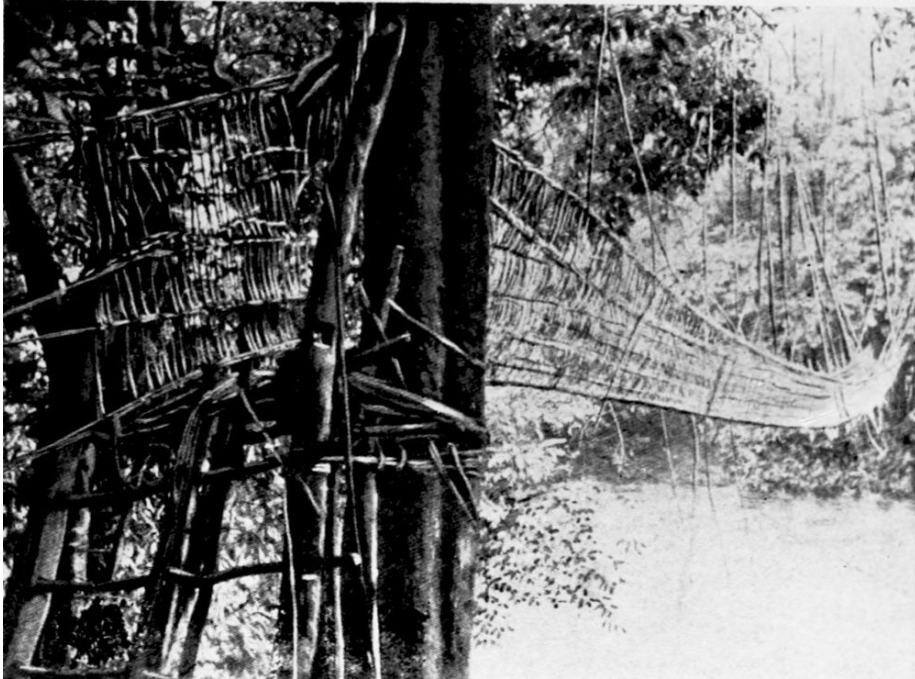
A SUSPENSION BRIDGE.
